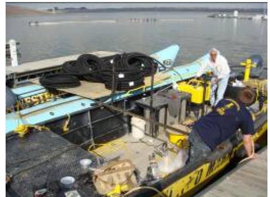
Inland Marine installing air lines and diffusers
