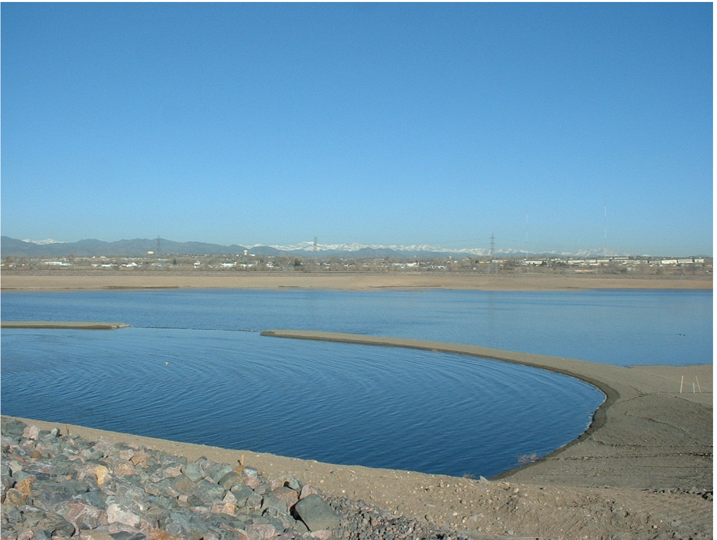
View of South Tani Reservoir Partially Filled Summer of 2006
