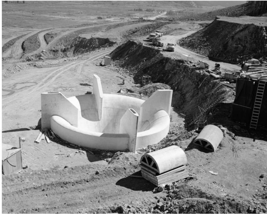
Crews work on building the reservoir's "Morning Glory" spillway, which discharges water into the Blue River downstream of the dam.
