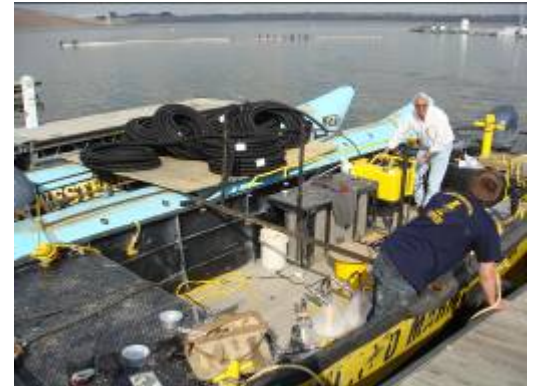
Inland Marine installing air lines and diffusers
